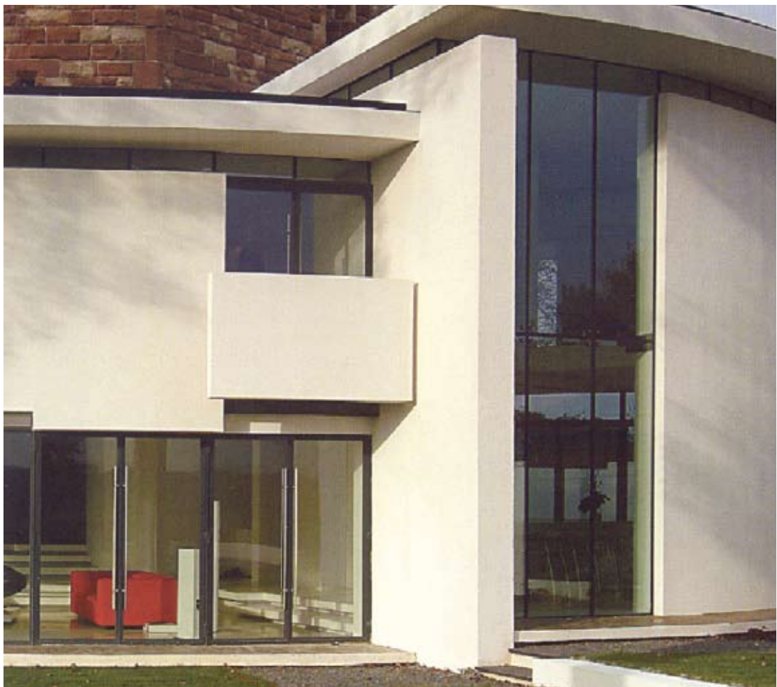
Lymm Water Tower, Cheshire Architect and building owner – Ellis Williams. System designer – Alumasc Exterior Building Products Ltd. Installer – Pegasus Externals Ltd.
