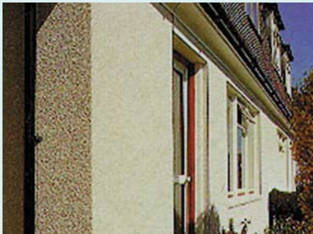
Figure 16 Example of a refurbished low-rise building
