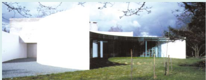
Figure 14 Example of a new build low-rise building – Crescent House, Wiltshire, by Foster and Partners
