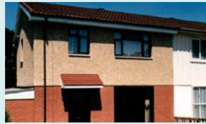
Figure 12 Example of a refurbished low-rise building – BISF housing, by Rugby City Council
