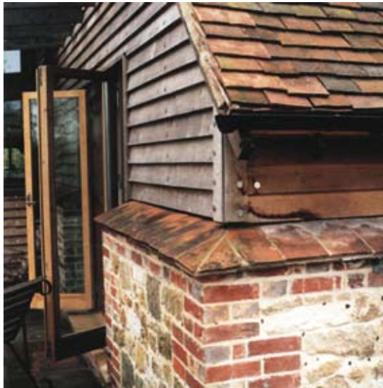
Figure 8 Bespoke system using unseasoned oak cladding, by Gale and Snowden Architects (Photo courtesy of Clive Boursnell)
