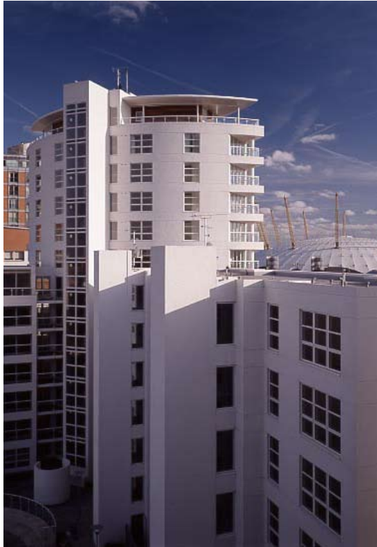
EWI system supplied by weber building solutions, architects: Goddard Manton, photography: Brauer Associates
